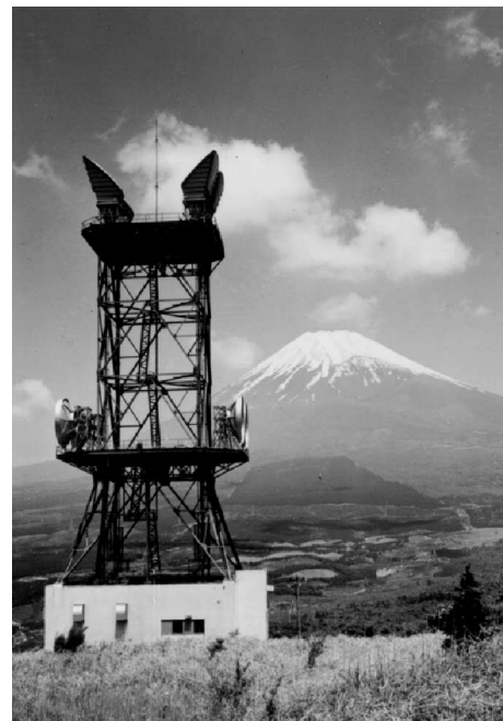
Fig. 7 Horn reflector antennas on the tower.
