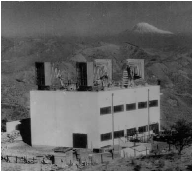
Fig. 2 Path-length lens antenna installed on a telephone building.
