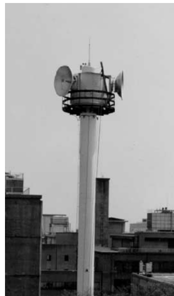
Fig. 15 Cassegrain antennas for 20-GHz band relay link.
