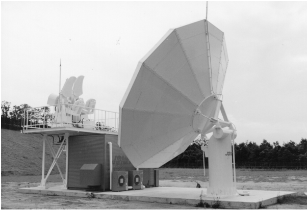
Fig. 13 Offset spherical reflector antenna at Osaka Teleport.
