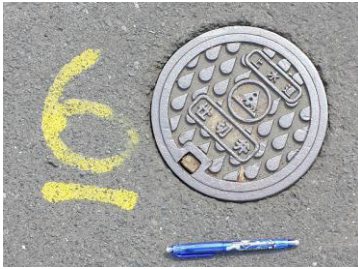
Fig. 11 External appearance of valve box.
