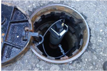
Fig. 12 Sensor terminal and internal appearance of valve box
